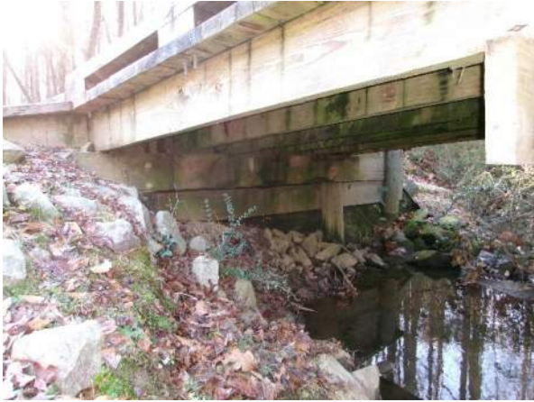
Typical of Bent 5 (looking ahead)
