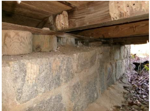
Typical of substructure members on top of masonry wall foundations
