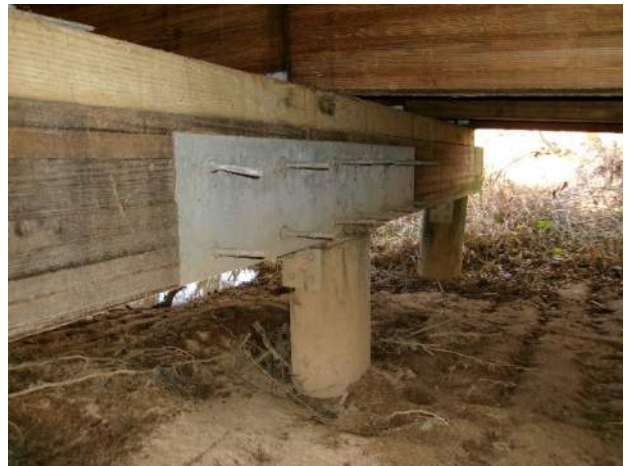
Typical of intermediate bent cap splice over Pile 2
