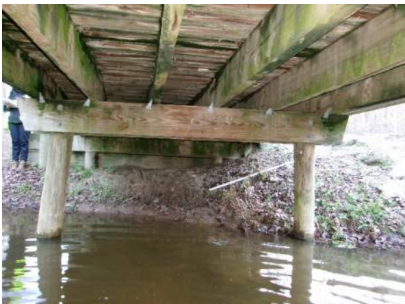
Typical underside (looking back)
