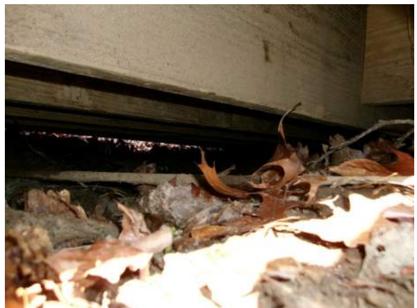
Typical underside (looking ahead)
