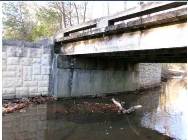
Bent 2 abutment has been encased in concrete and wing walls added
