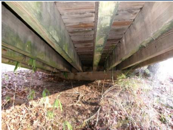
Typical underside of bridge (looking back), Bent 1 piles are below grade
