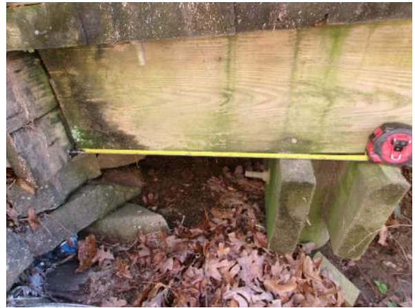
Span 1 overhanging Bent 1
