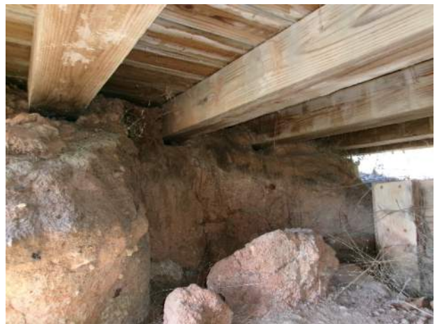
Typical of abutment and endroll
