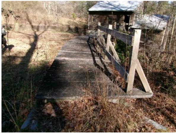
Topside of timber approach and handrail
