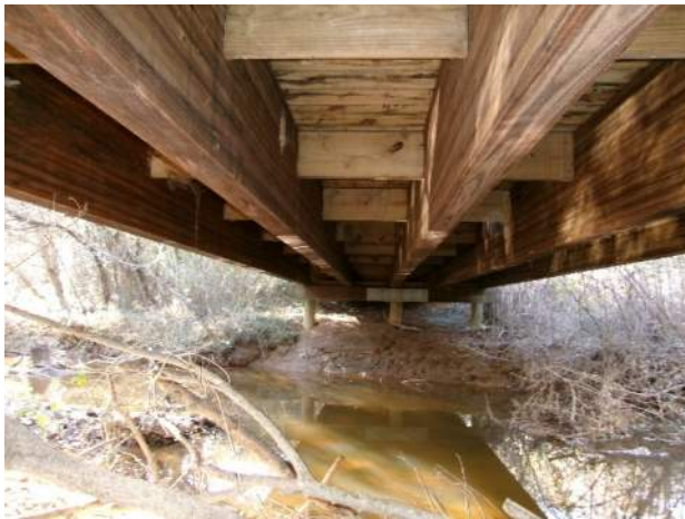
General underside (looking back from Bent 3)
