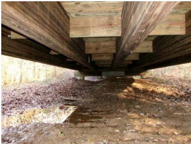
General underside (looking ahead from Bent 2)
