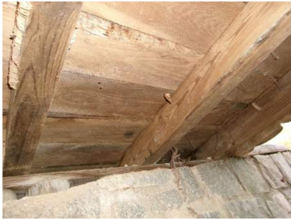
Typical of bottom of decking and superstructure
