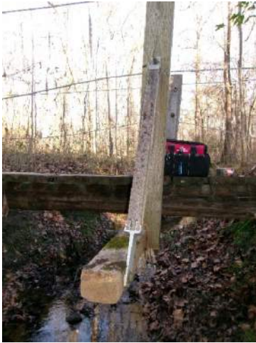
Typical of vertical handrail post and kicker support
