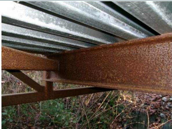
Typical protective coating patina of steel members under the bridge deck
