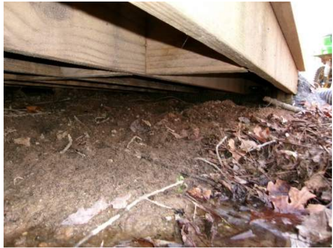
Typical underside (looking back)
