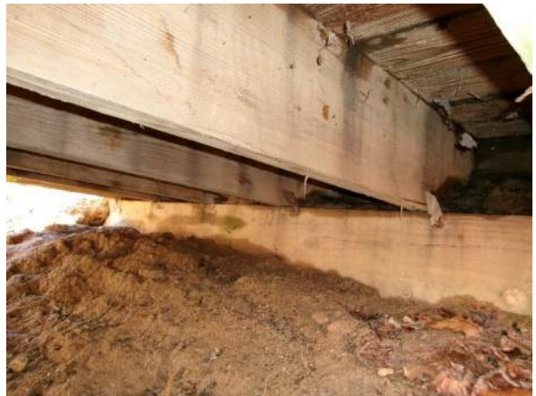
Typical end bent (Bent 2 shown)
