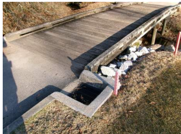
New drop inlets and rip rap added to Bent 5
