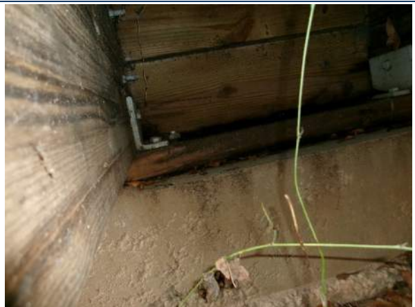
Typical of 3"x8" mud sill and beam connections using steel angles
