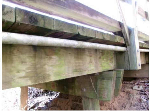
2" diameter PVC utility along right side of bridge deck
