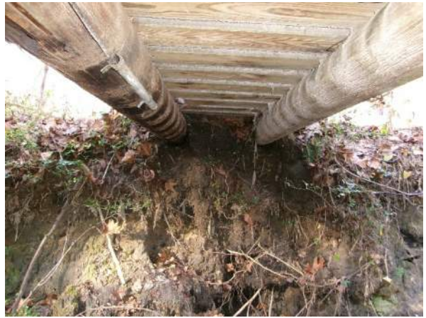
Typical underside (looking ahead)
