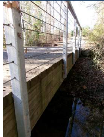
Typical of handrail connection to exterior beams (looking back)
