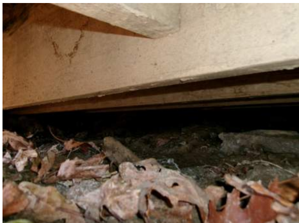
Typical underside (looking back)
