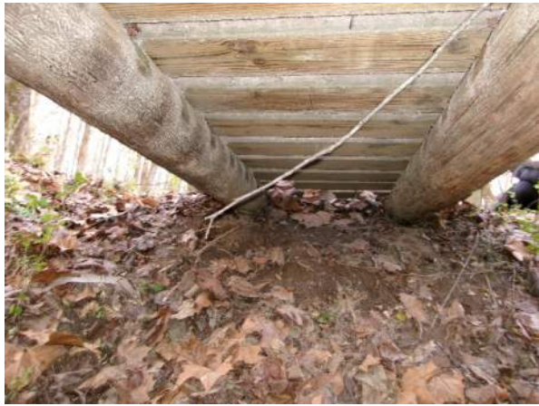
Typical underside (looking back)
