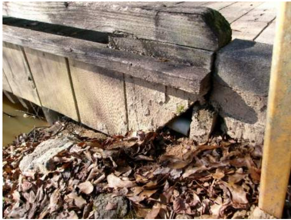
Timber façade covering 2" diameter PVC utility
