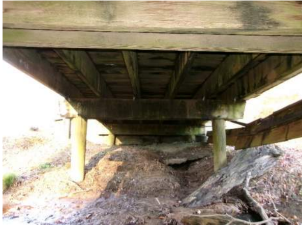
Typical bridge underside (looking back)
