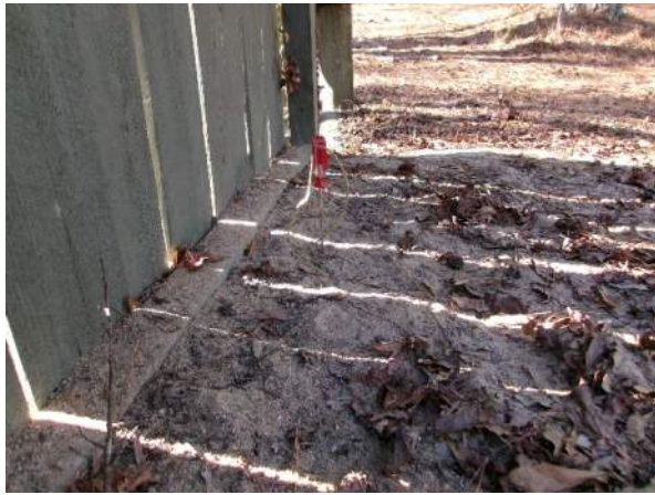
Typical of dirt along deck
