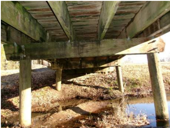
Typical underside of bridge (looking back)
