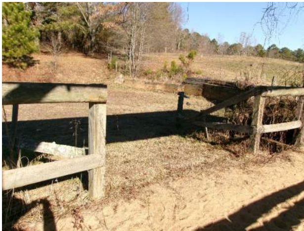
Dirt ramp tie-in to bridge deck
