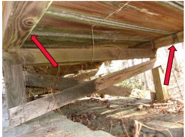
Typical of superstructure, deck boards supported by 4"x4" stringers (looking ahead)
