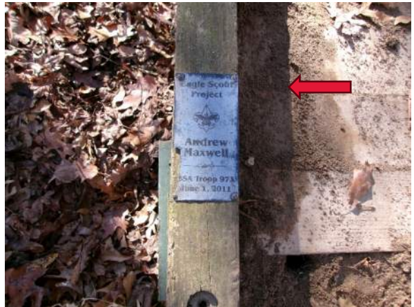
Structure date of construction marker
