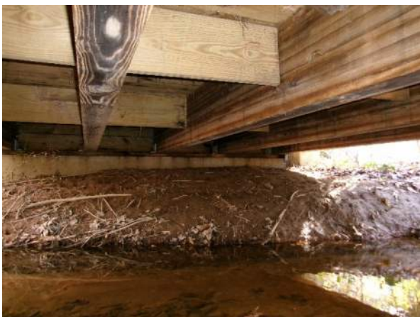
Typical underside of bridge (looking ahead)
