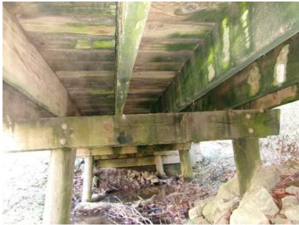
Typical underside of bridge (looking ahead)
