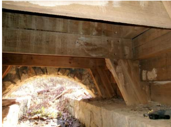
Typical underside of timber culvert (looking downstream)
