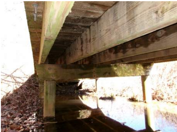
Typical underside (looking back)
