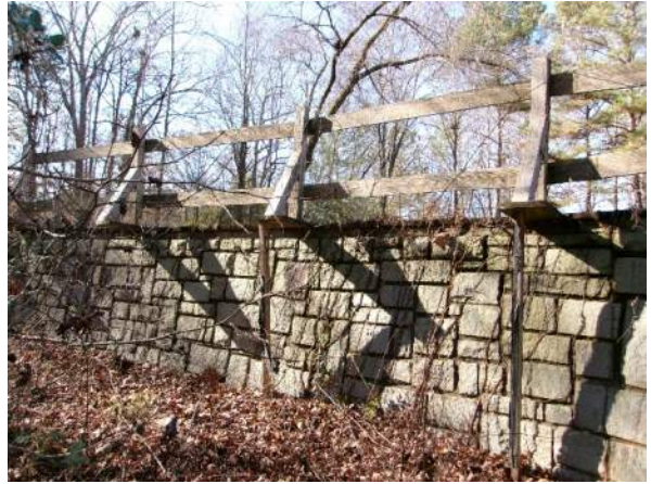
Handrail of timber approach with 2"x4" kicker braces
