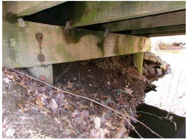
Typical end bent (Bent 4 shown)
