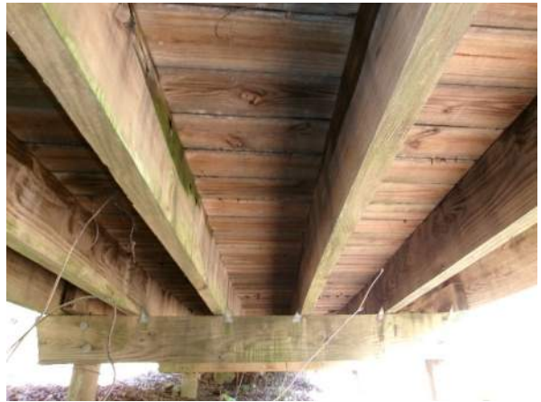
Typical bridge underside (looking ahead)
