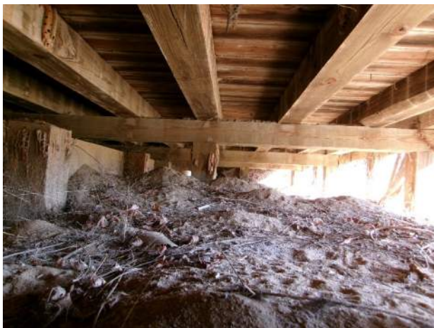
Typical underside of bridge (looking ahead)
