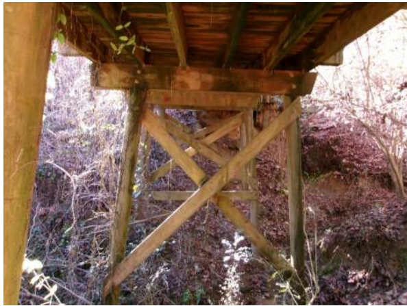
Typical underside of bridge (looking ahead)
